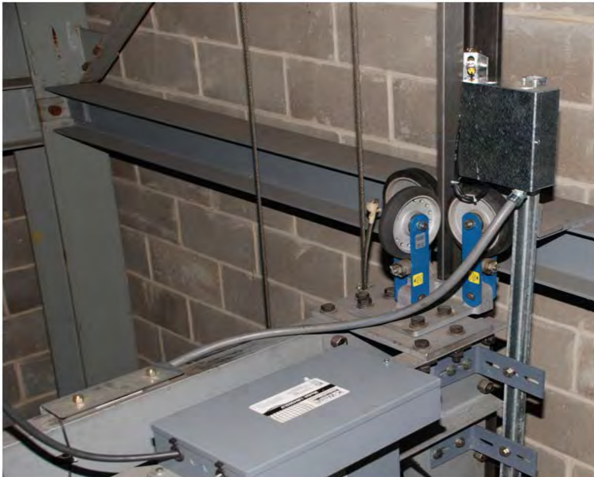
Figure 2.5: Tapeless Selector Mounted on Crosshead
